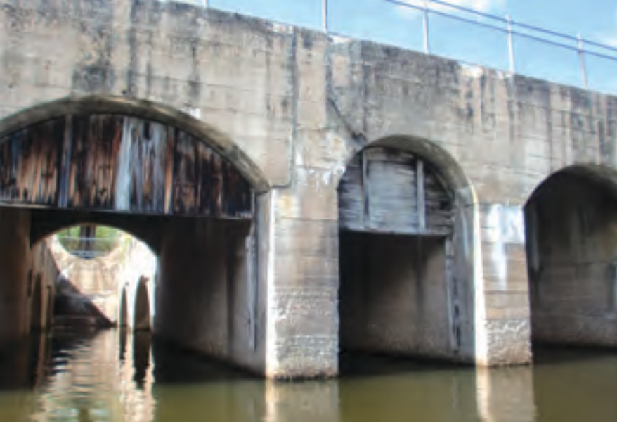
View of Old Pinawa Dam from water.
