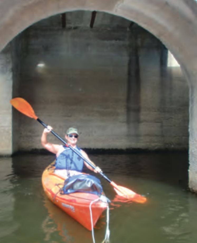
Lise Boiteau paddling under Old Pinawa Dam structure.
