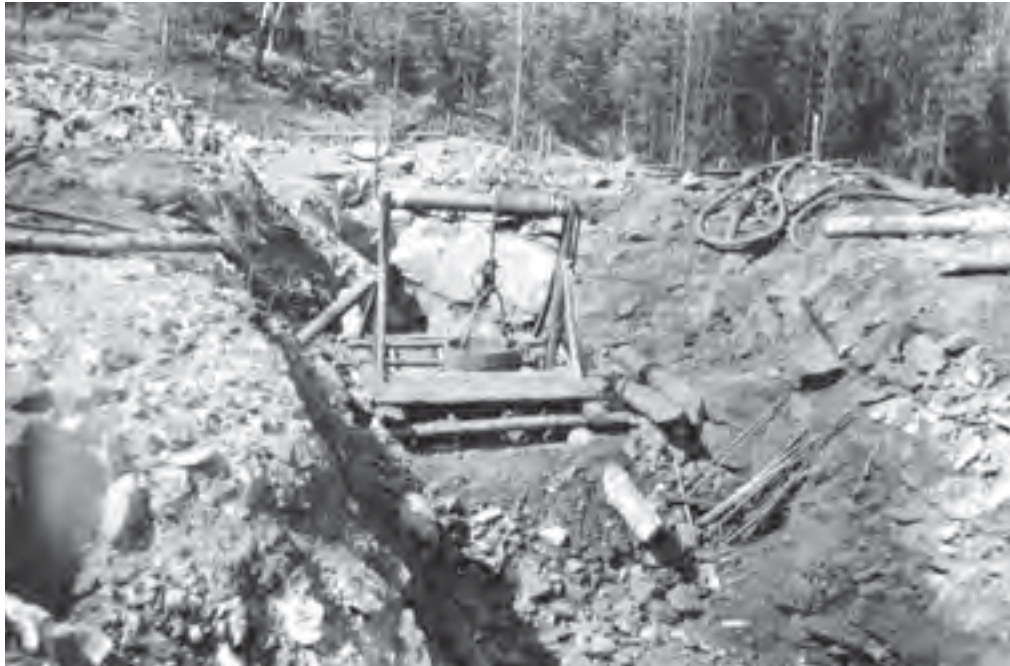
Early mine shaft construction.
