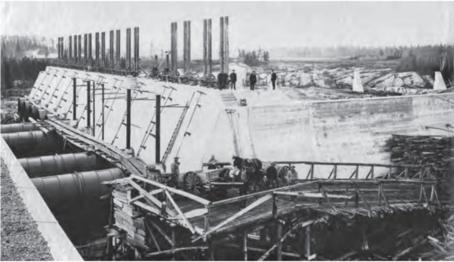
Pinawa generating station construction Credit: Friends of Old Pinawa
