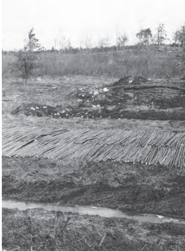
Corduroy over muskeg with drainage ditches Credit: History & Folklore of the Whiteshell Park South
